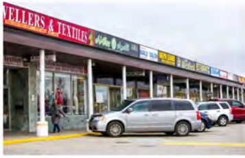
Neighborhood Service Center
